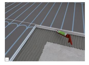
The wedi PreLine is laid across the full surface with a thin-bed mortar (recommendation: wedi 320 universal tile adhesive) and aligned. In wet areas, the building board joints must be fully and thoroughly bonded and sealed with wedi 610 adhesive sealant (recommendation: one bead of wedi 610 underneath the milling groove and one bead level with the milling groove).
