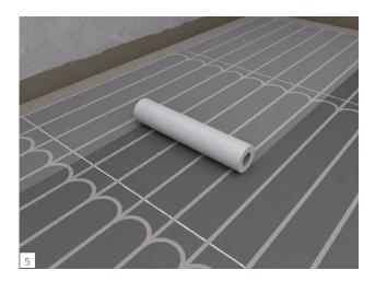
The entire surface must be covered with 600 mm wide, selfadhesive reinforcement tape (recommendation: wedi Tools 600 mm joint reinforcement tape).
