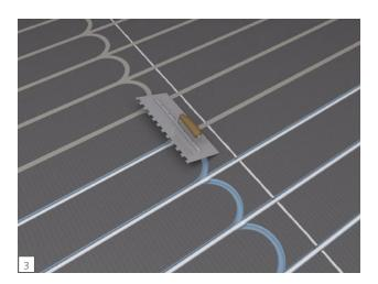
Lay pipes in the groove. Backfill the pipe ducts with tile adhesive, e.g. wedi 320 tile adhesive.
