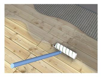
It is important for the surface on the wooden beam coating to be properly implemented before installation of the wedi PreLine system is begun.
