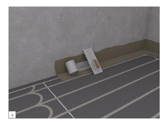
In wet areas, the building boards / wall connections must be implemented with a sealing tape using a liquid sealant (recommendation: wedi Tools sealing tape with wedi 610 or wedi 520). All intersections in the wedi PreLine must be properly sealed.
