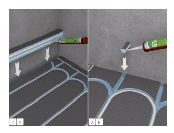
In wet areas, the open ends of the groove in the edge areas of the wedi PreLine must be waterproof.
