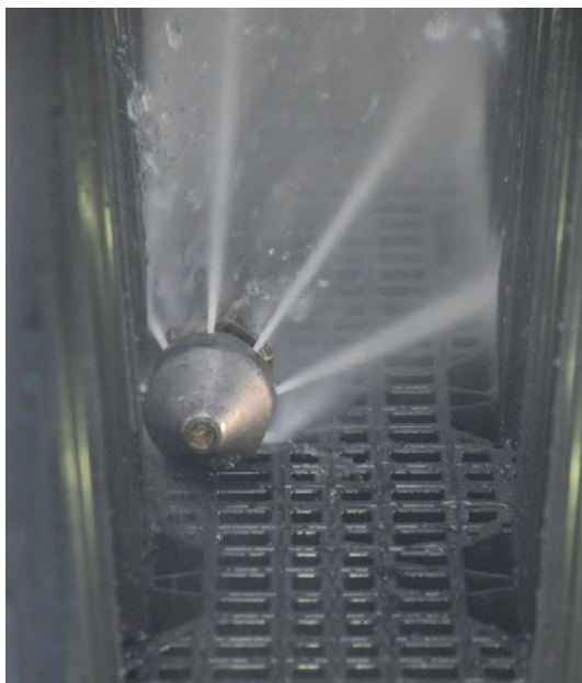
Figure 12 - Jetting nozzle flushing the system
