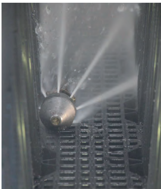
Figure 8 - Jetting nozzle flushing the system
